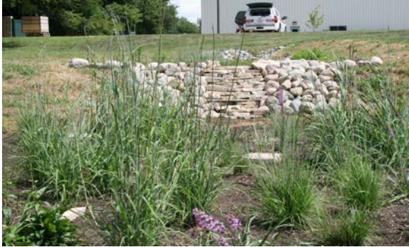
(a) Cascading feature in two-stage bioretention cell at the Coralville Fire Station.
