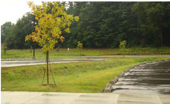
(c) Newly planted bioretention area in Ames with native grasses.
