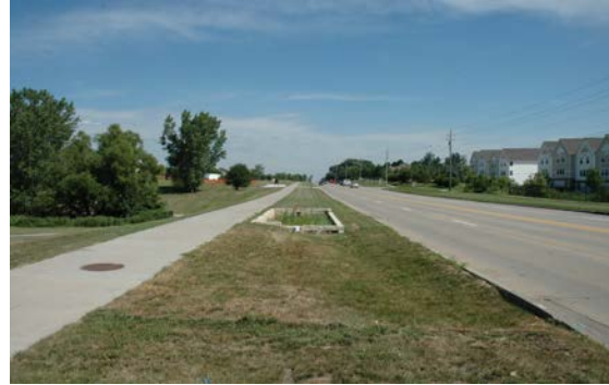
(b) The grassed pretreatment area provides a long flow path to this bioretention cell in Ankeny. Curb cuts were installed after the young plants became established.
