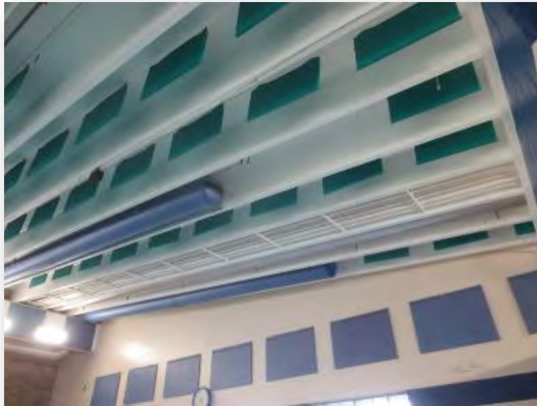
Lap Area – View Looking North
