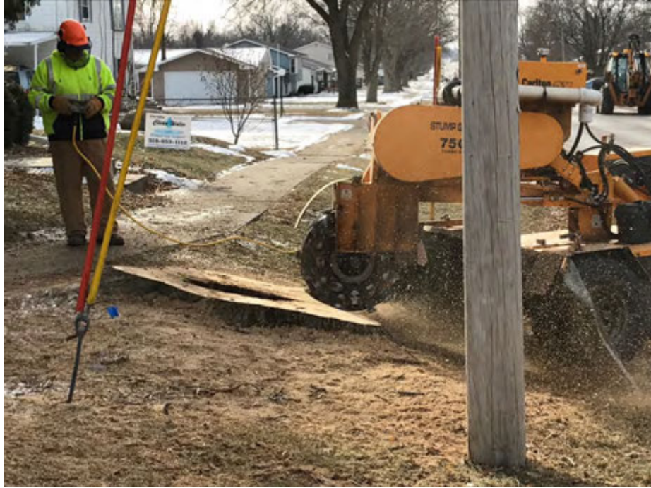
Large trees and stumps removed for N Front St construction project
