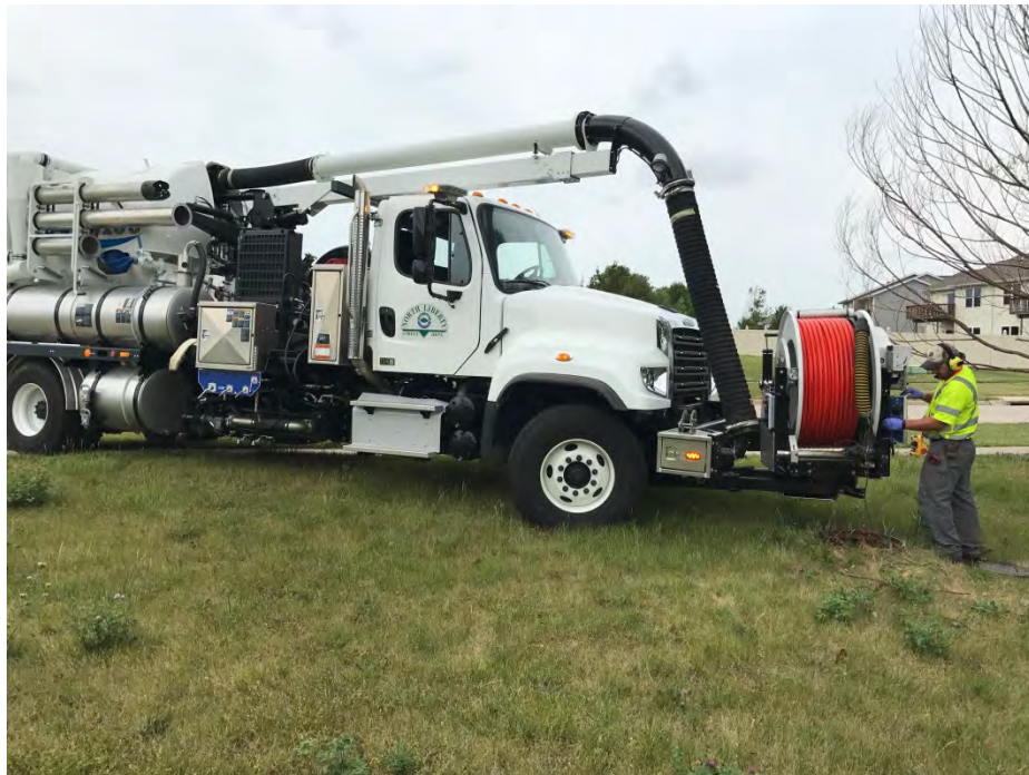
Sanitary sewer jetting and vacuuming process
