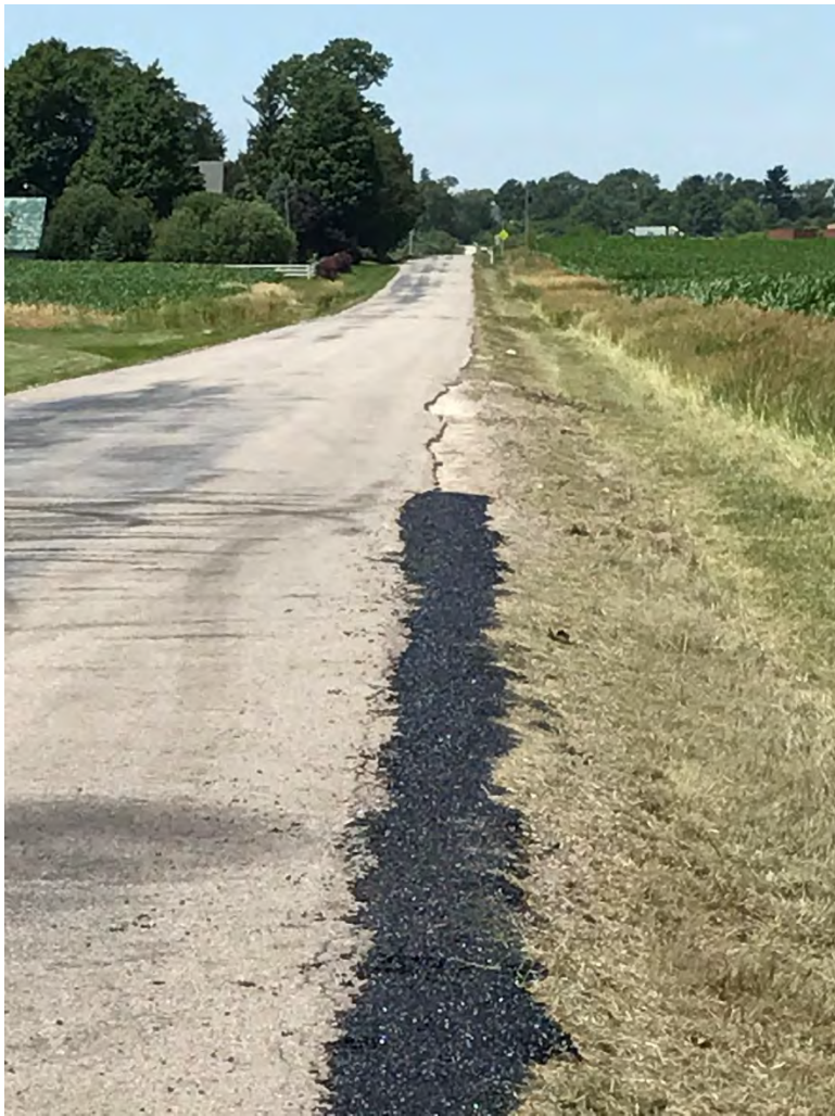
St Andrews Drive shoulder repair in process
