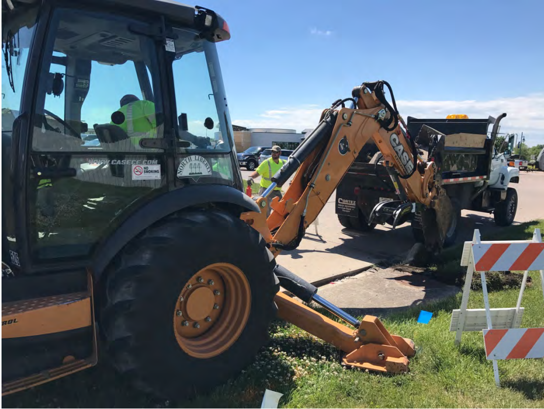
Concrete panel replacement
