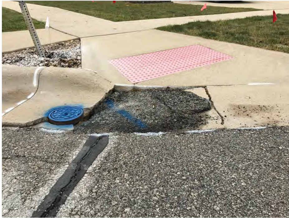
Concrete curb and street had failed.
