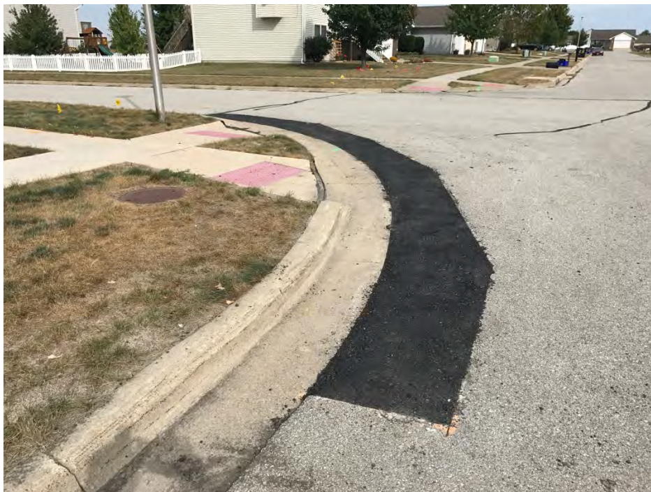
Smooth transition after repair.
