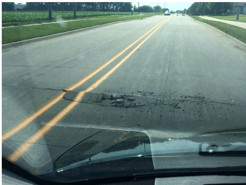
Concrete "Blow up" because of heat
