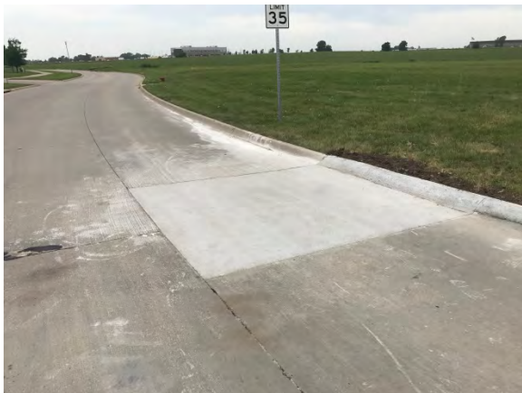
Concrete "Blow up" because of heat
