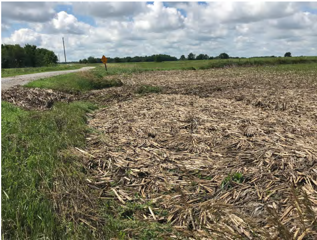
Corn stalk debris plugging drainage pipes
