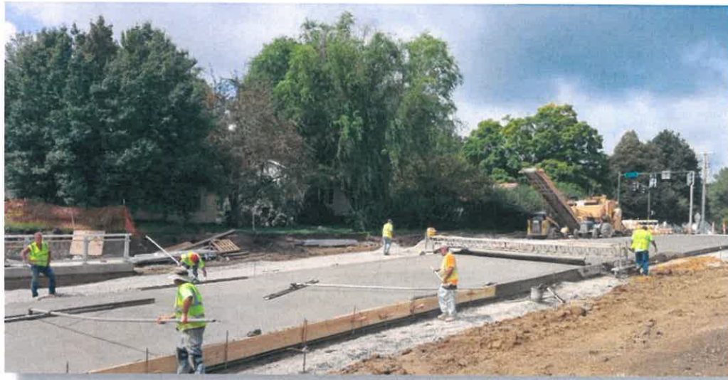
Reconstruction of First Avenue for grade separation under the Iowa Interstate Railroad.
