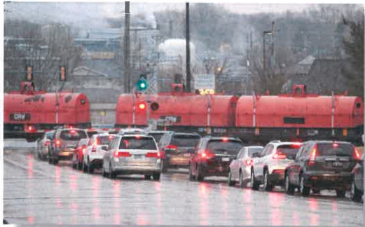
Prior to the construction of the First Avenue railroad overpass in Iowa City, traffic congestion and delay was a significant issue along this important north-south corridor in Iowa City.
