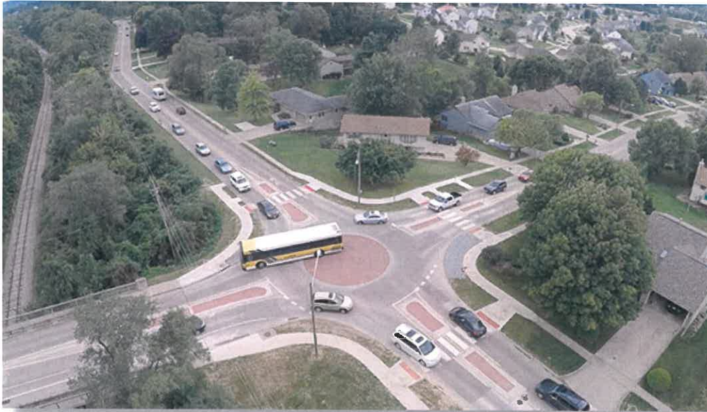
A roundabout at 12th Avenue and Holiday Road in Coralville has reduced congestion and travel delay at this busy intersection.
