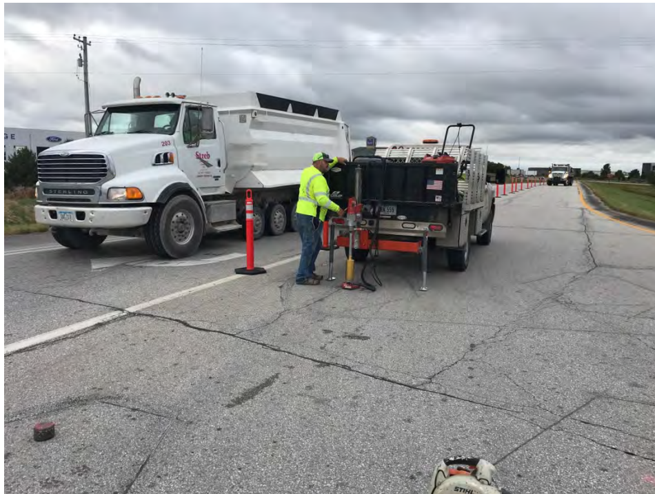
Installation of Adaptive Traffic hardware on I380 exit ramp
