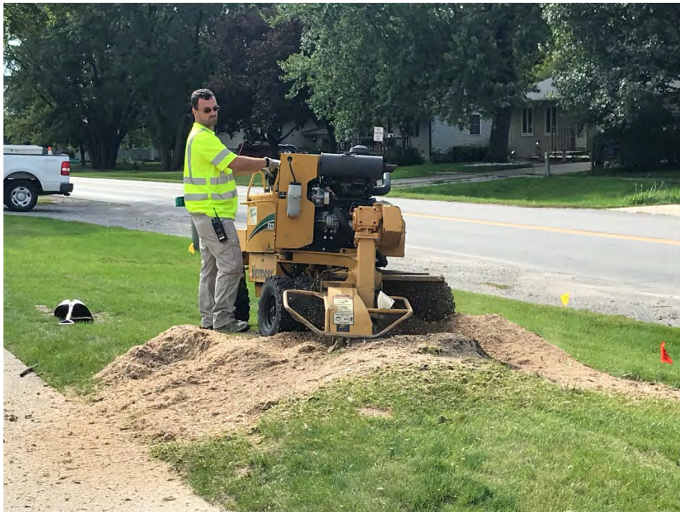
Stump grinding of City trees removed in the right of way
