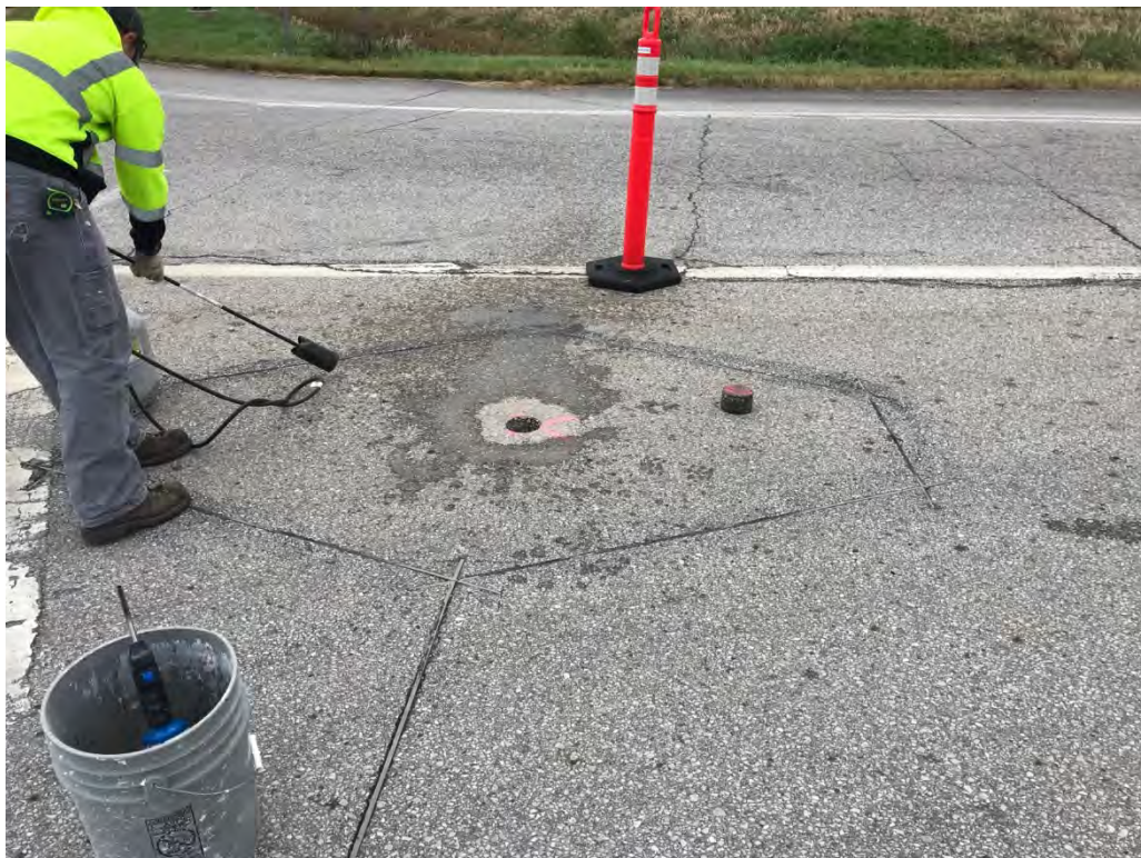
Preparing surface for detection hardware install for Adaptive system
