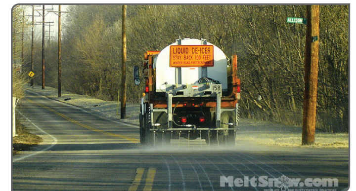
Anti-icing streets before a snow or ice storm. MeltSnow.com
