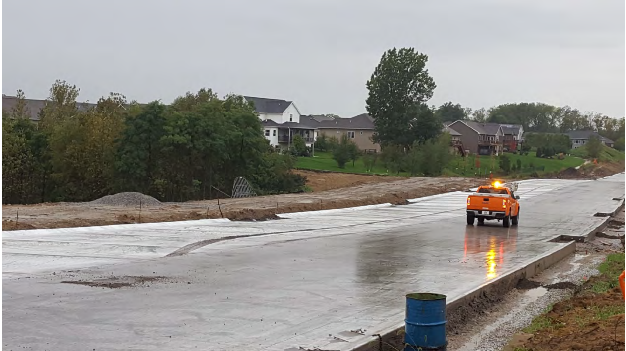
Forevergreen Rd damaged sections
