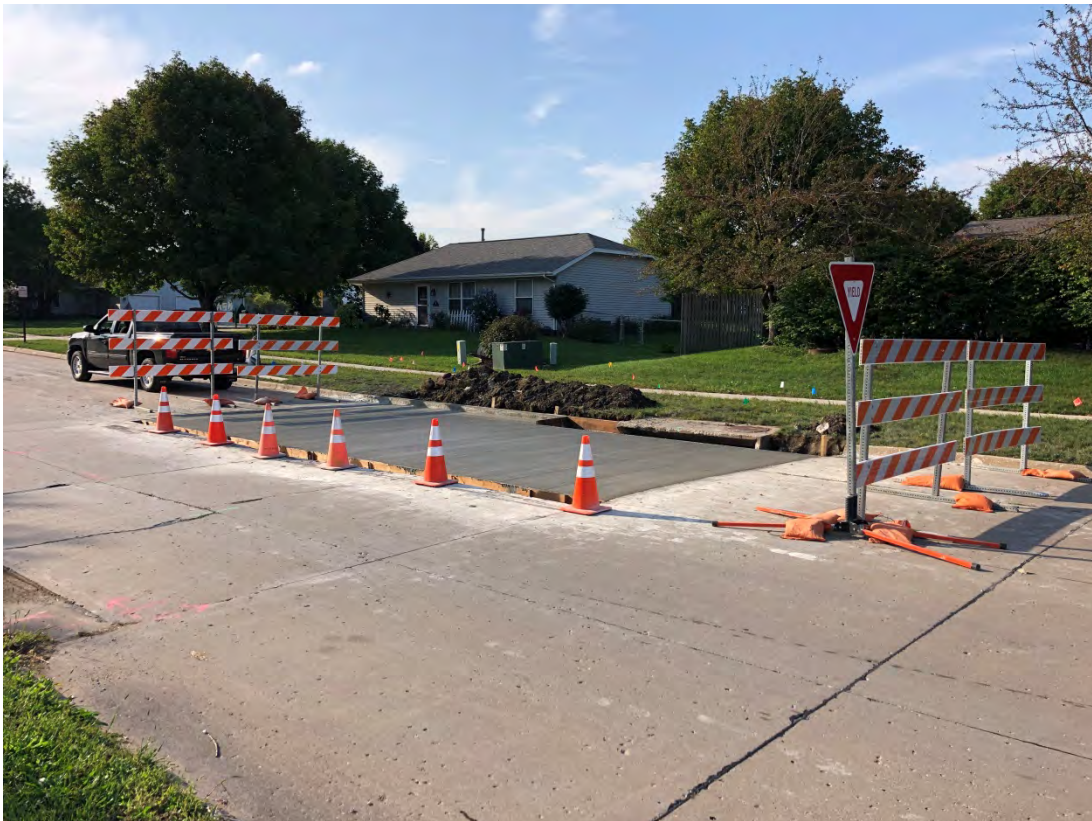
West Zeller Street repair
