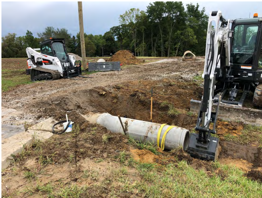
Storm pipe being installed for dog park driveway
