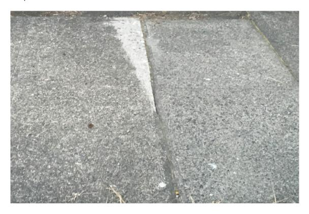
"Stub toes" are areas in the sidewalk, where part (or all) of one square is higher than the one next to it, causing a tripping hazard for pedestrians. It may be possible to eliminate the "stub toe" hazard by grinding down the high edge.
