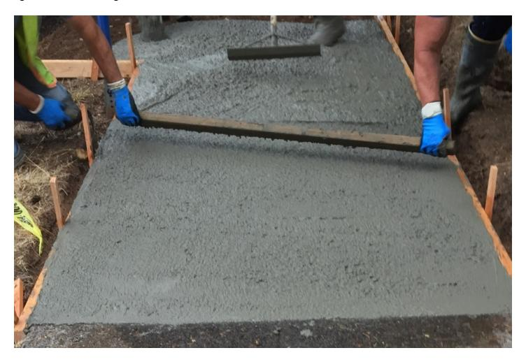
Next use the edge of a 2" x 4" board or "screed", that reaches across the entire width of the formwork and move it across the surface in a sawing motion. Concrete should be the same grade as the existing formwork, which should be at existing grade of abutting sidewalk.
