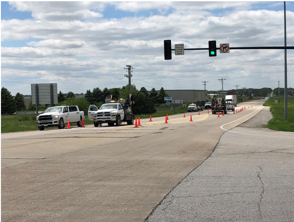
Street line painting on Penn Street
