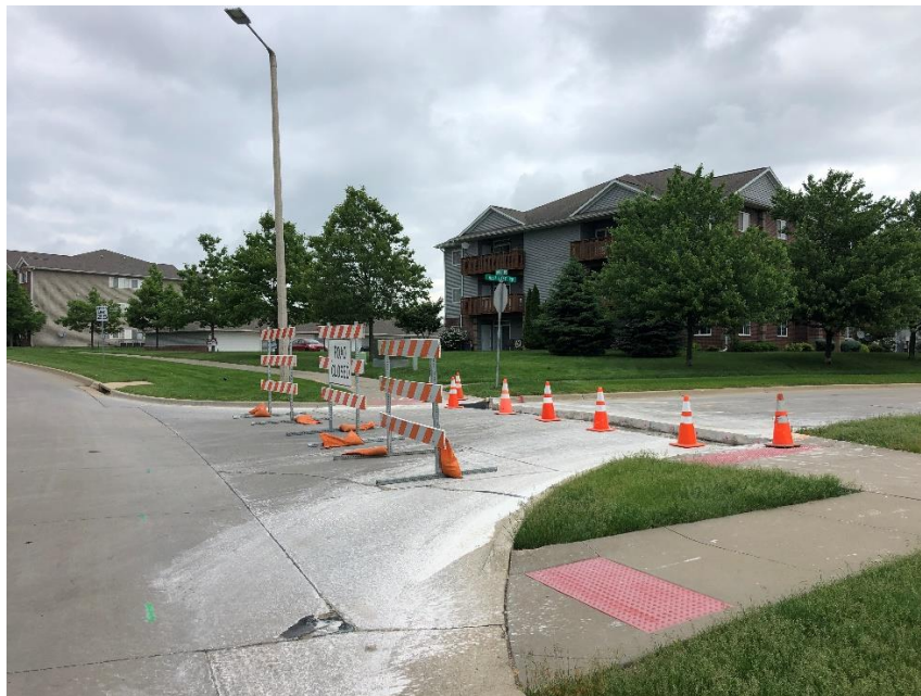
West Lake area street repairs
