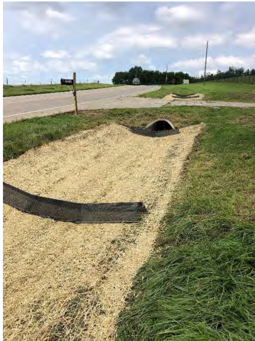
North Liberty Road erosion area restored
