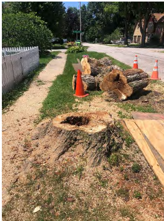
Large tree removals showing hollowed out base in right of way.
