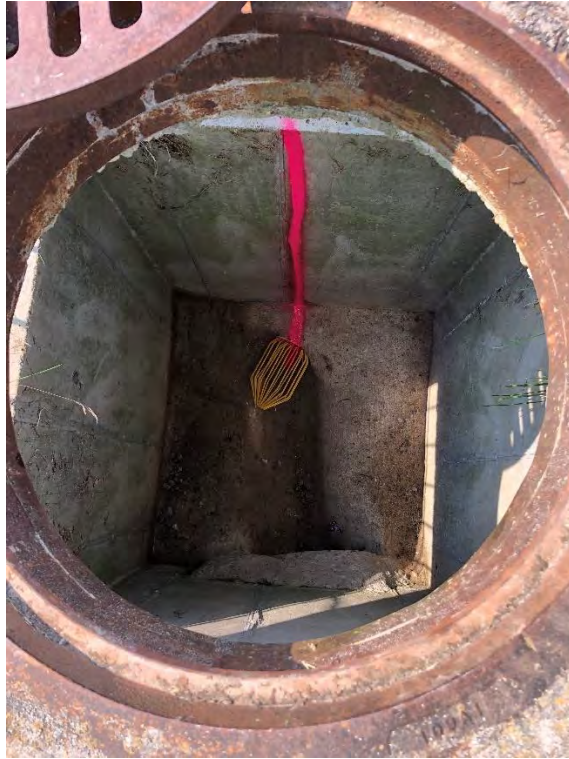
Windsor Farms storm drainage basin cleaned and improved guard system installed
