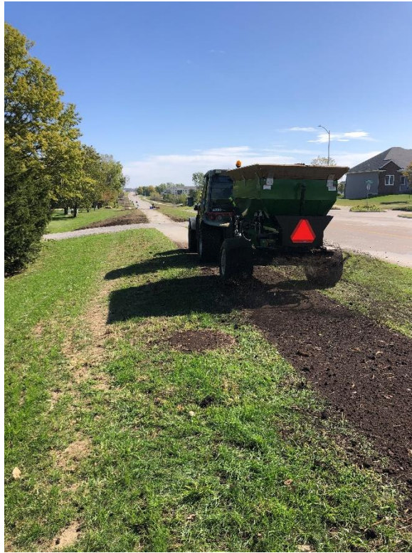
Installing compost material for West Forevergreen Rd 321 project
