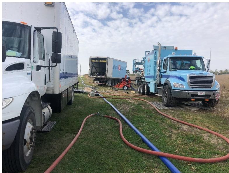
CIPP process for West Trunk Sewer Main
