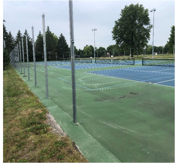
Beginning stages of the tennis court project.
