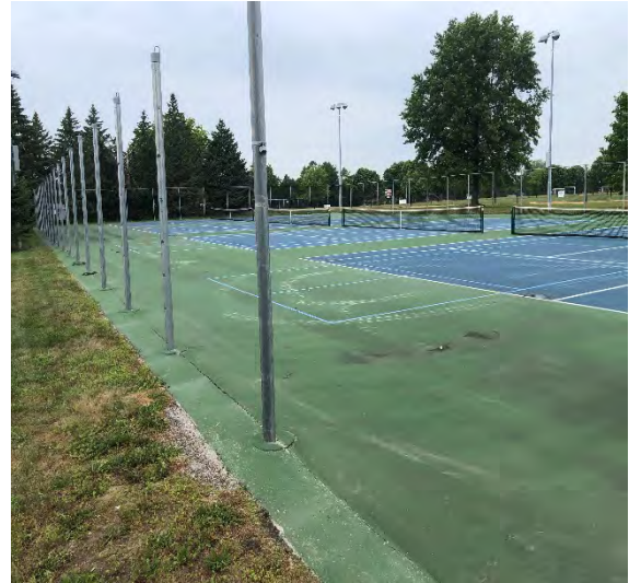
Beginning stages of the tennis court project.
