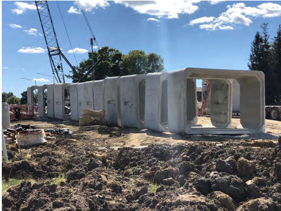
Pedestrian tunnel sections unloaded and staged for install
