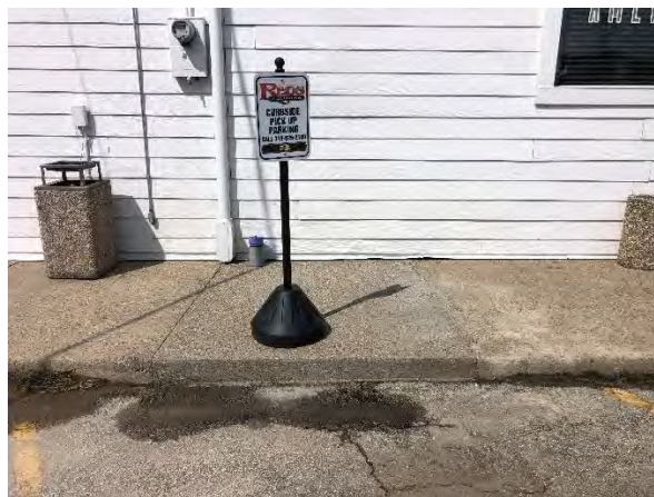
Staff removed and reinstalled matching concrete for Dubuque St Phase 1 electric
