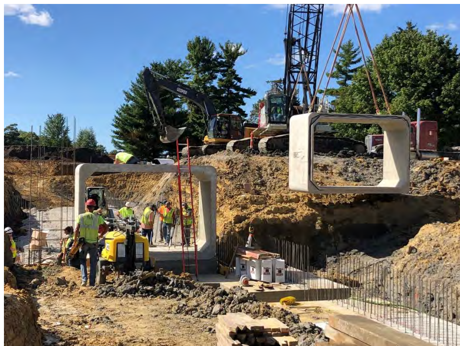
Tunnel sections being installed
