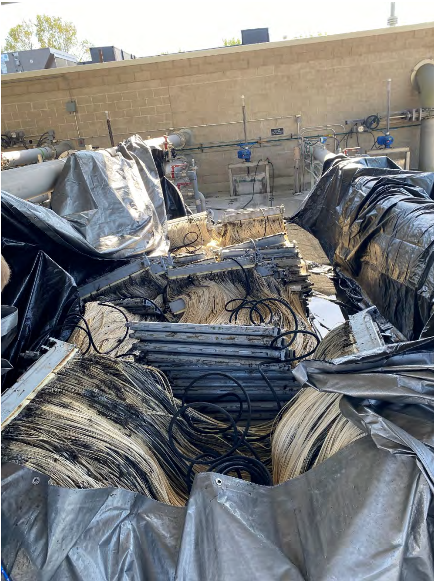
70 Modules saved for replacing in other trains
