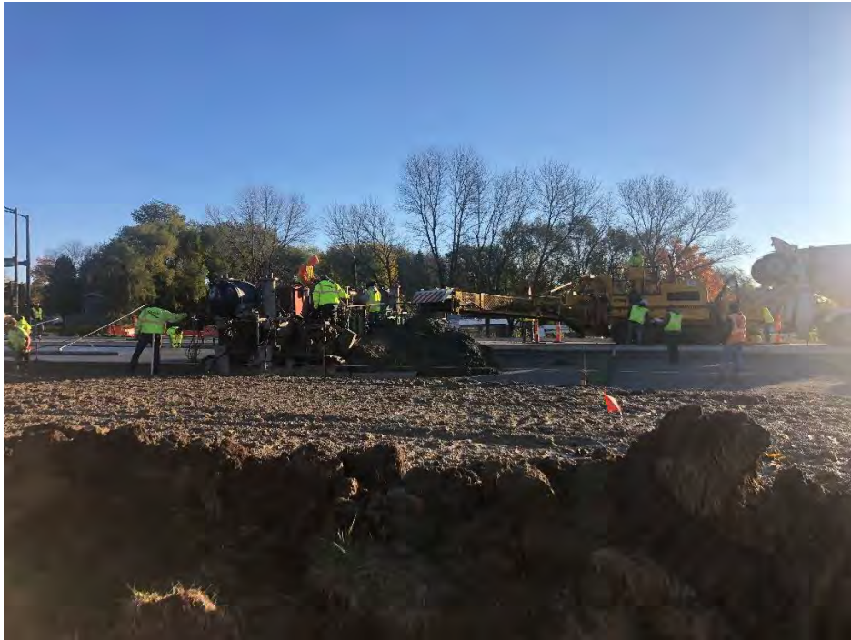
Ranshaw Way concrete pour on west side in front of Fareway
