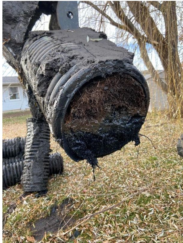
Storm pipe removed. Blockage from tree roots and trash debris. Repairs still continuing.
