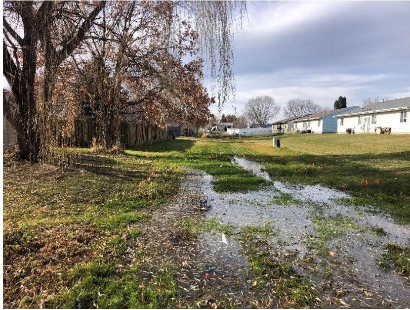
Sugar Creek Ln drainage blockage in backyards
