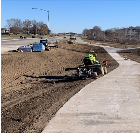
Park staff final grading along the Forevergreen Rd. Trail Project.
