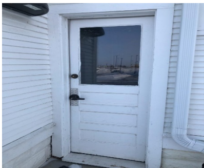
Ranshaw House door rebuild
