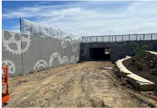
Ranshaw Way pedestrian tunnel anti-graffiti clear coat application by contractor.
