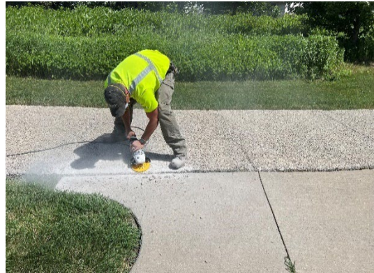
Concrete trail repairs.
