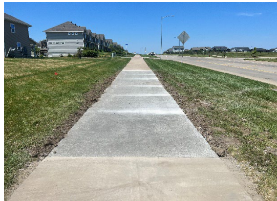
Concrete trail repairs.
