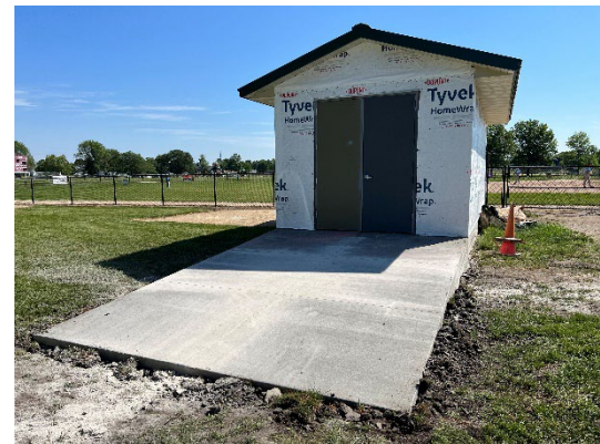
Babe Ruth shed received a new steel standing seam roof, steel doors and a concrete ramp.
