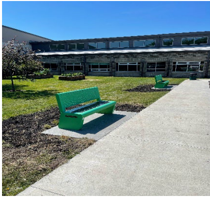
Concrete pads and benches installed.
