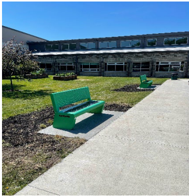
Concrete pads and benches installed.
