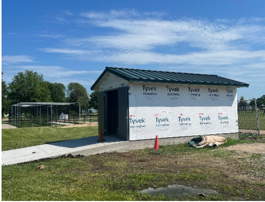
Babe Ruth shed received a new steel standing seam roof, steel doors and a concrete ramp.
