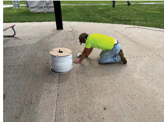
Concrete crack sealing at Penn Meadows Park.
