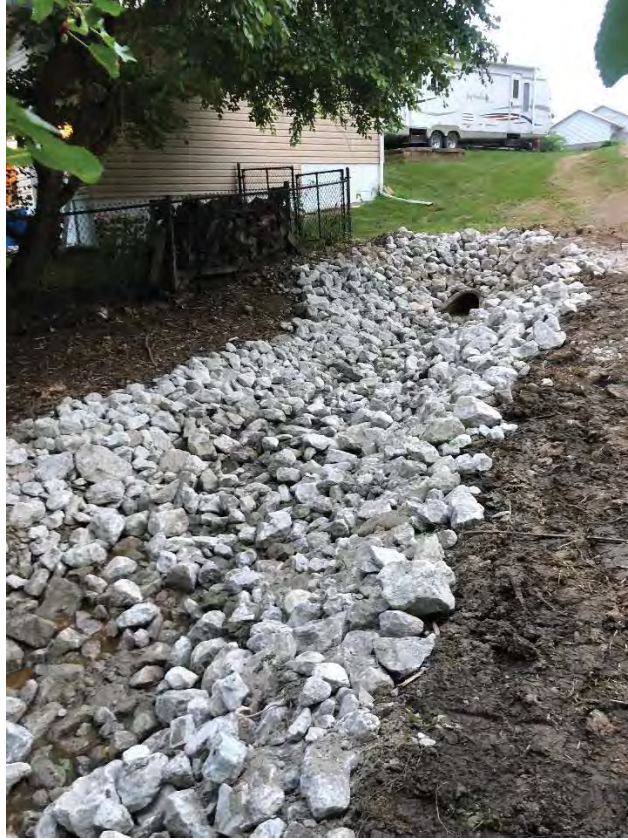
Storm repair work completed by staff before and after picture
