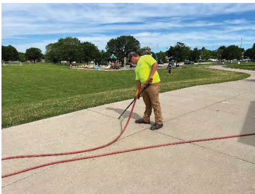
Concrete crack sealing at Penn Meadows Park.
