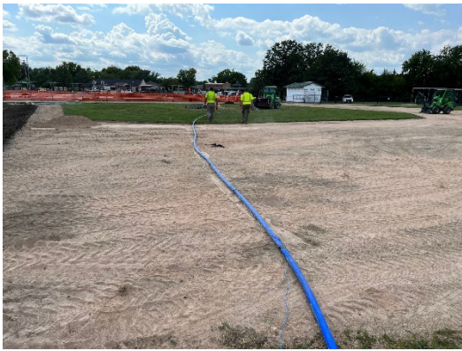
Water line, back flow preventer and meter install at the Babe Ruth baseball field.
