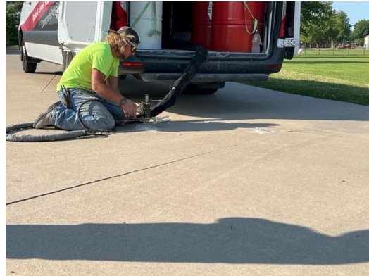
Concrete lifting to eliminate trip hazards at Penn Meadows Park.
