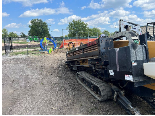
Water line install at the Babe Ruth ball field.
