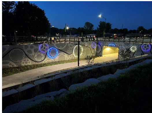
New pedestrian tunnel aesthetic wall lighting.
