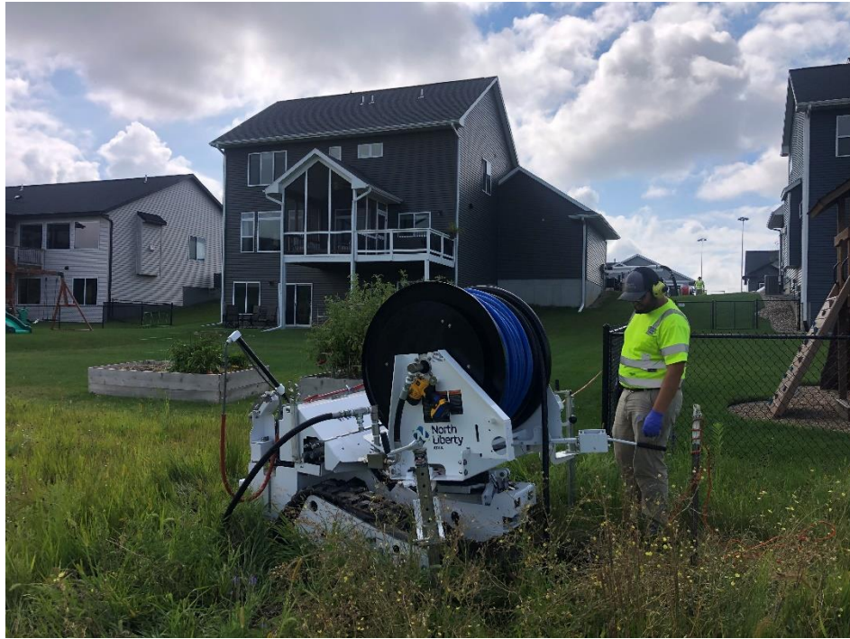
Jetting sewers in remote locations with easement machine
