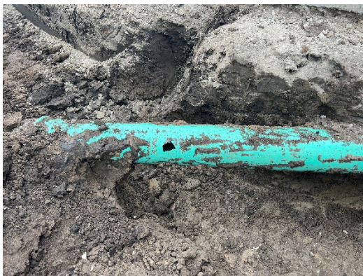
Sewer line repair at the Babe Ruth building.
