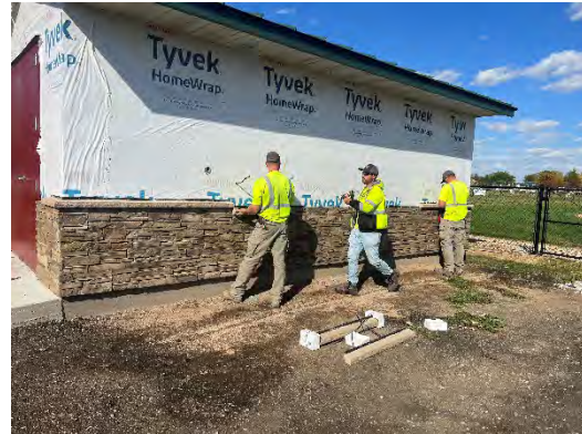
Park staff at Babe Ruth field installing brick and siding on the new shed.
