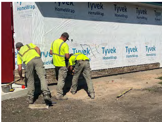
Park staff at Babe Ruth field installing brick and siding on the new shed.
