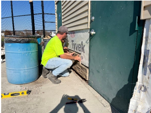
Park staff at Babe Ruth field installing brick on the press box/restroom facility.
