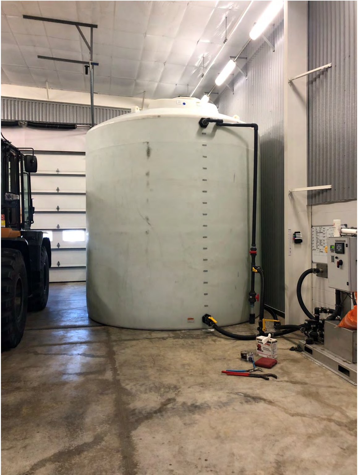
Installation complete on 10,000-gallon brine storage tank
