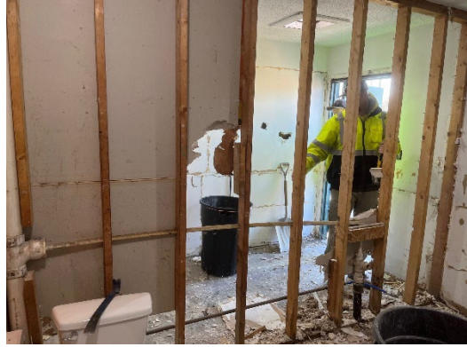
Demolition work on the interior Babe Ruth building.
