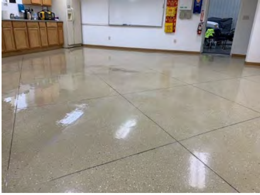
Resurfacing of floors at the Parks facility.
