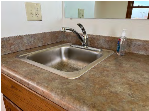
Facuet replacement at the Ranshaw House.
