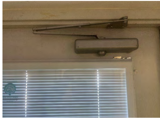
Door closures adjustments at various locations.
