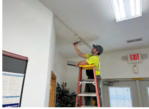
Drywall repair at the Parks facility.
