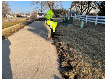
Snowplow turf damage repair in multiple locations along trails.
