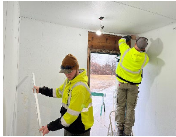
New wall board installation at the Babe Ruth press box facility.
