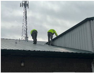
Parks facility leaky roof repair.
