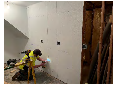
New wall board installation at the Babe Ruth press box facility.
