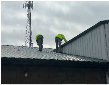
Parks facility leaky roof repair.
