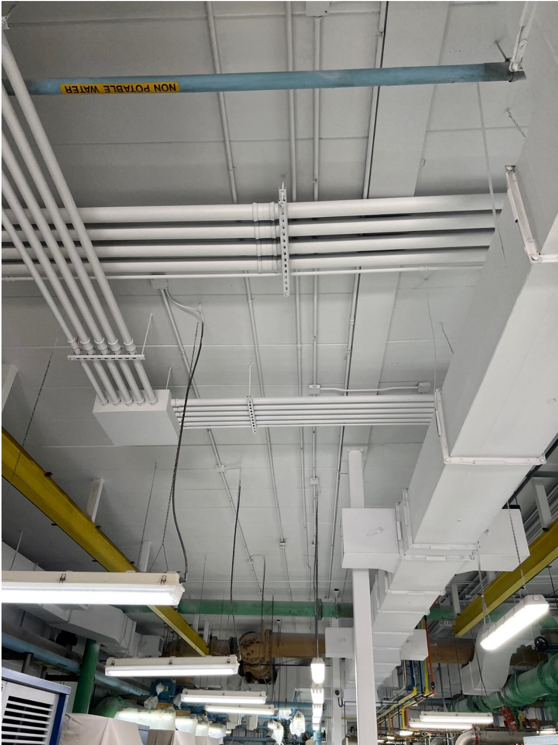
CEILING, WALLS, CONDUITS, AND DUCTING REPAINTED
