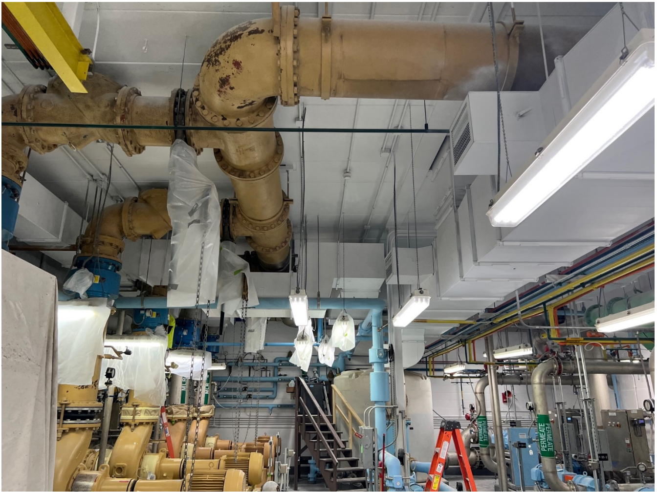
PROCESS PIPING PREP WORK
