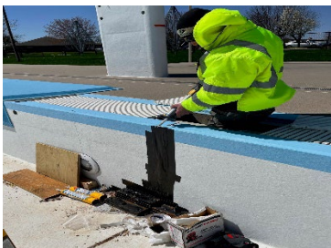
Outdoor Pool wall repair.
