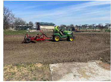
Dubuque Street Project final grading near Penn Elementary and the Babe Ruth Field.
