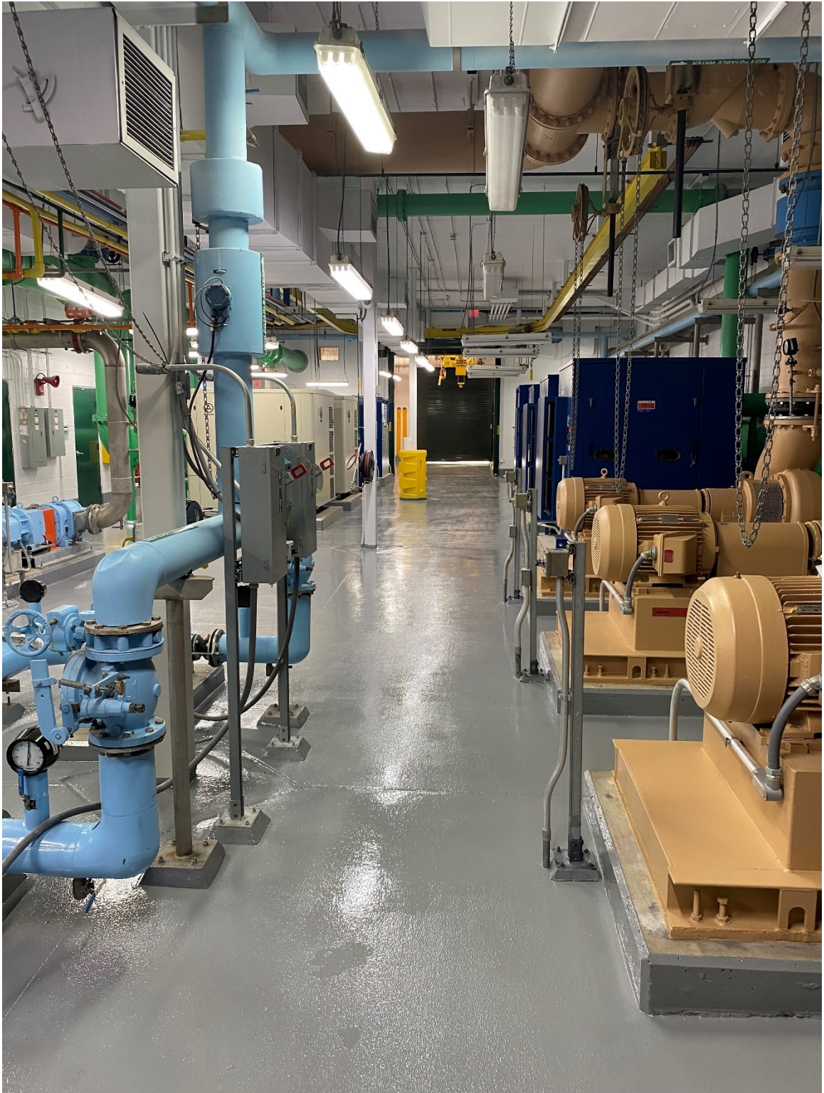
Piping and Equipment Repainted
