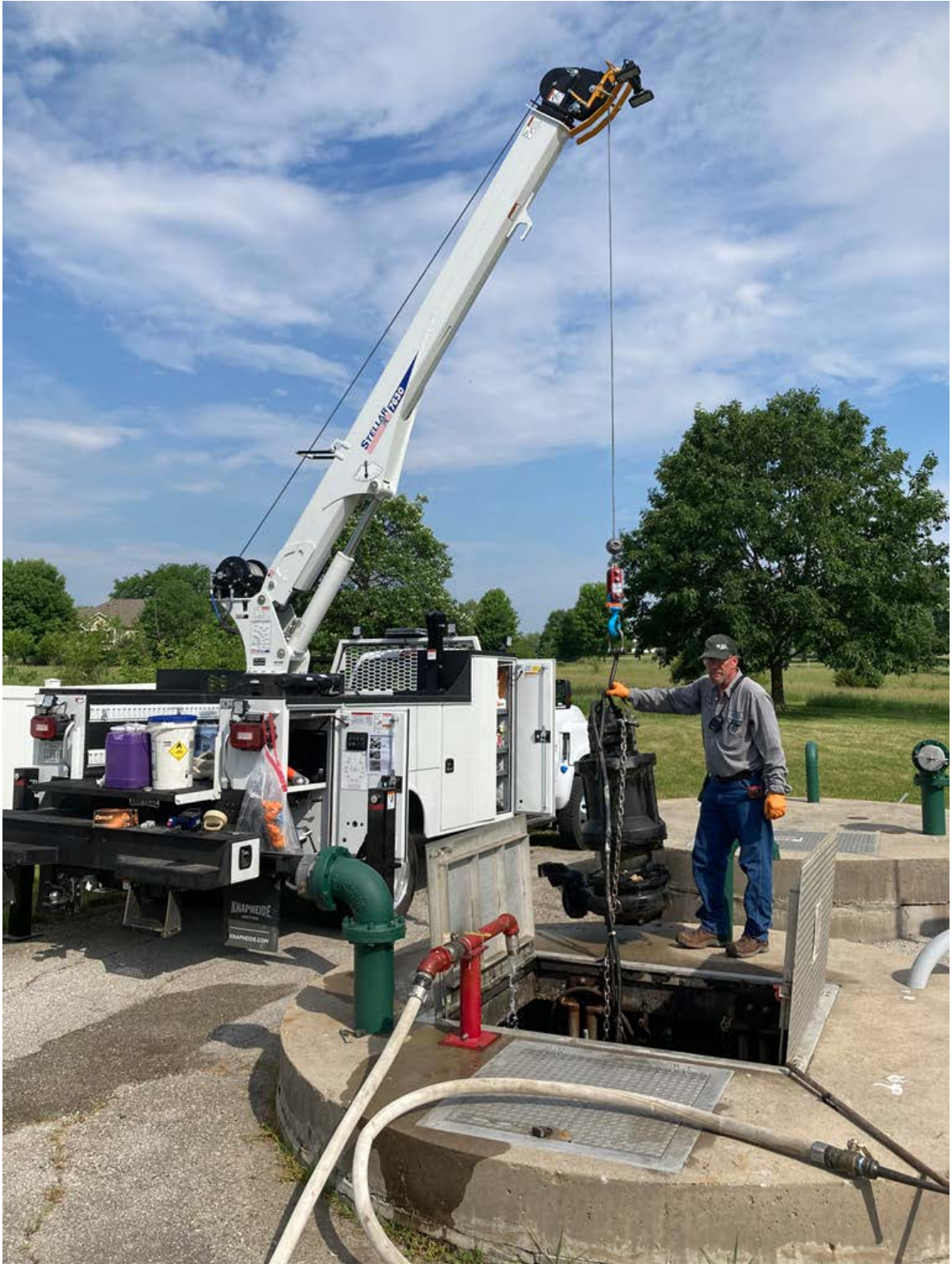
New Crane Truck Pulling Submersible Lift Station Pump (Cedar Springs)
