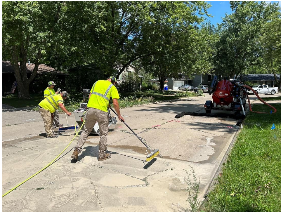
Heritage St prep for removals and replacement
