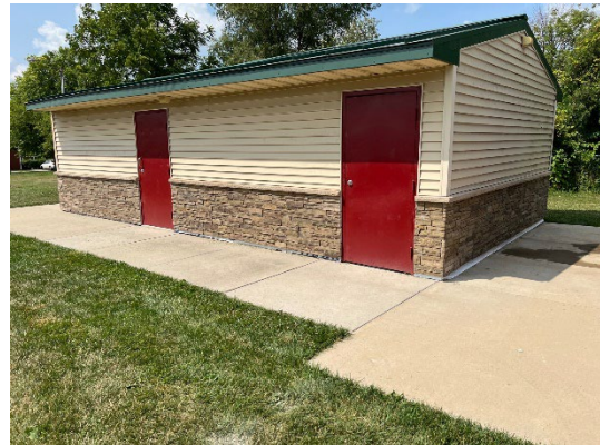
Koser Park building stone veneer and siding completion by the Parks Department
