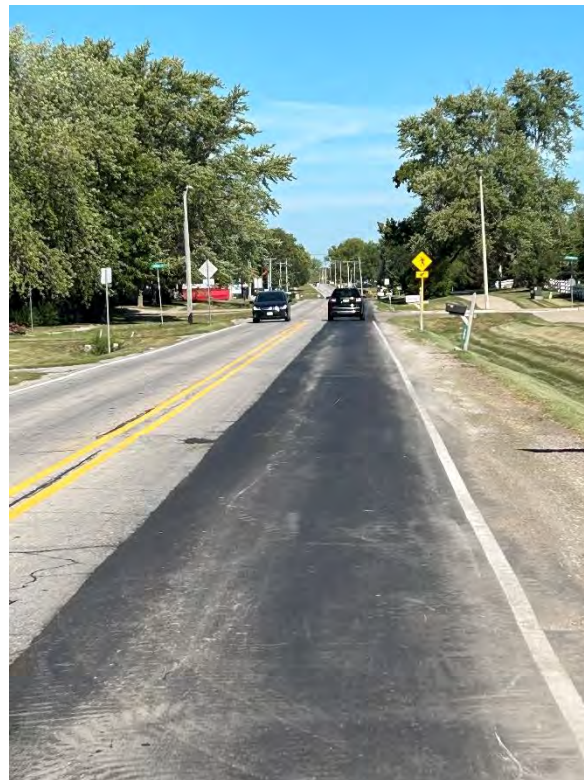
South Dubuque St asphalt repair
