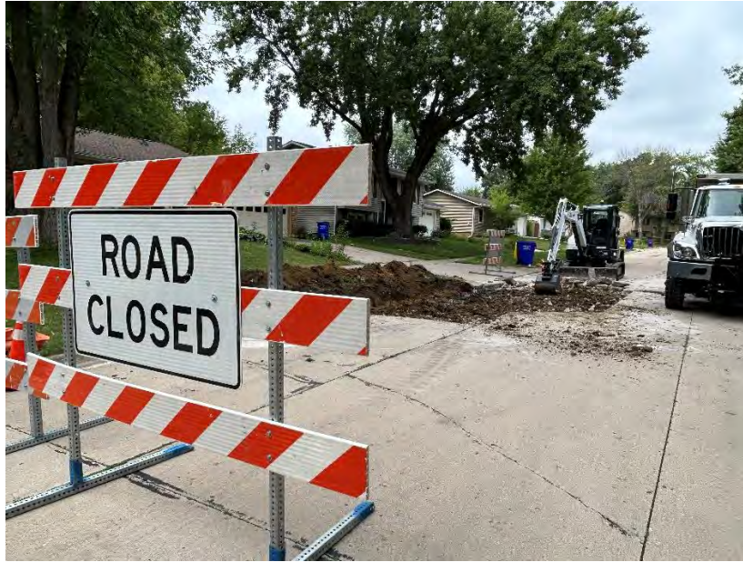
Street repairs on Heritage Dr
