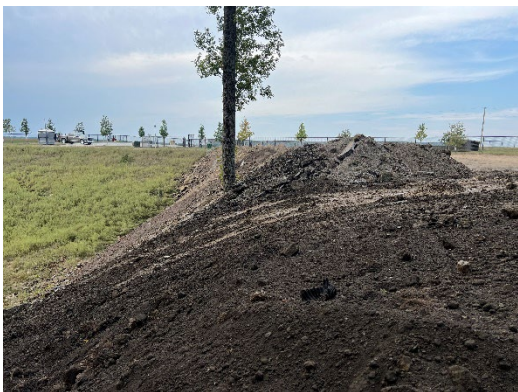
Fill dirt from the Penn Meadows Parking lot project used at Red Fern Dog Park for berm addition and enhancement.
