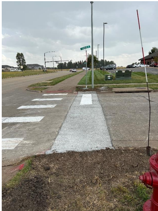
Lininger Ln repairs
