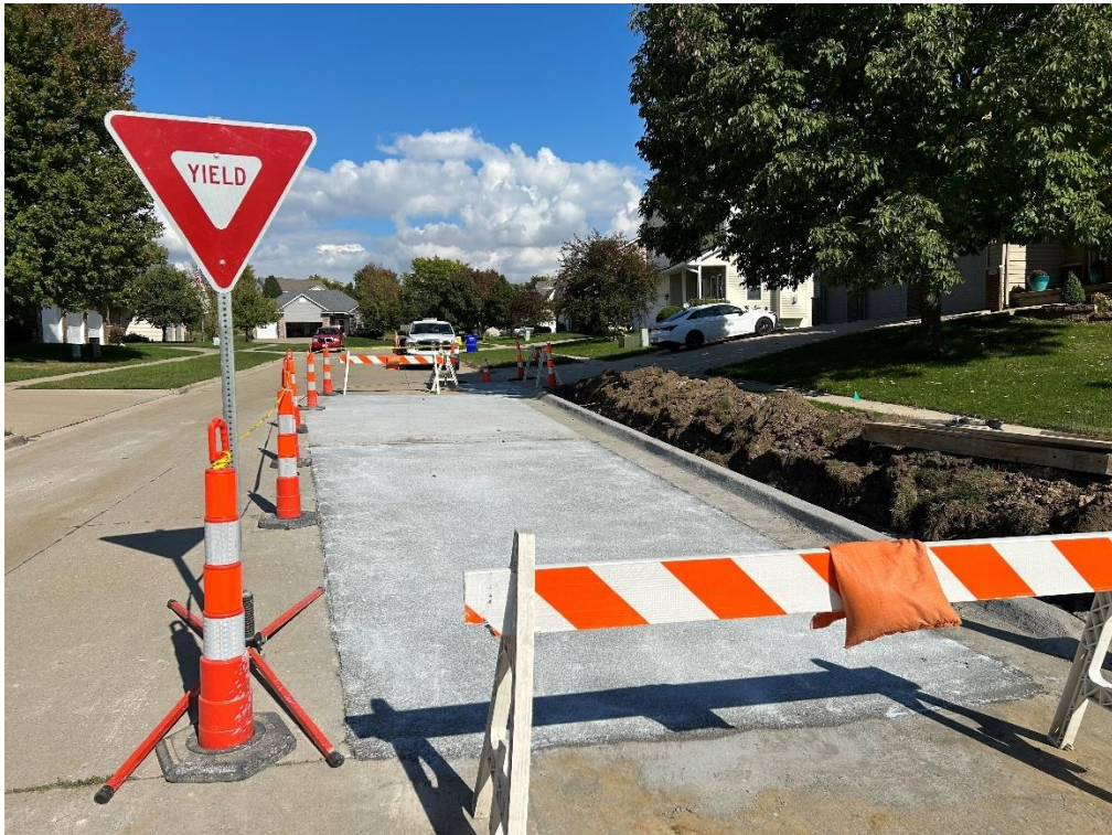
Willow Ln repairs
