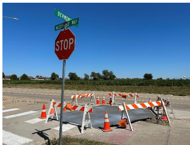
Devmont Ct repairs
