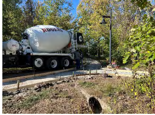
Cornerstone Park concrete trail removal and replacement.
