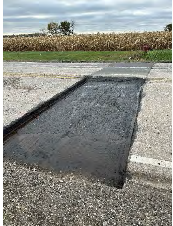
Milling bump location on South Dubuque St and then resurfacing with hot asphalt mix
