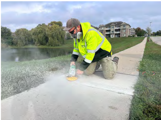
Annual trail & sidewalk trip hazard grinding.
