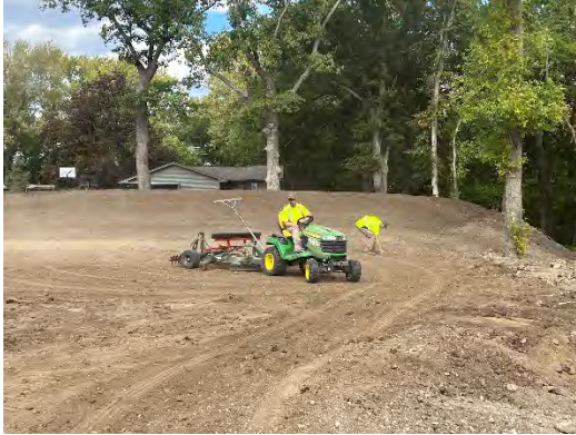
Red Fern Dog Park berm grading and seeding.
