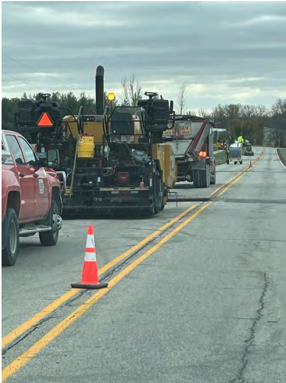
Milling bump location on South Dubuque St and then resurfacing with hot asphalt mix
