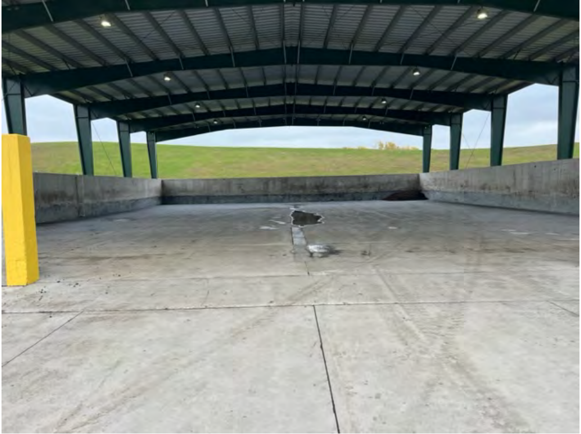
Biosolids Storage Bld. Cleaned and Drains Flushed
