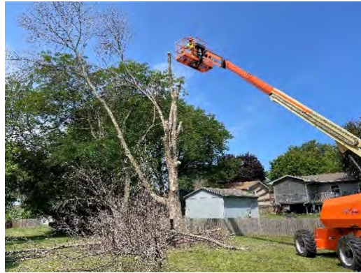
Tree removal continues.
