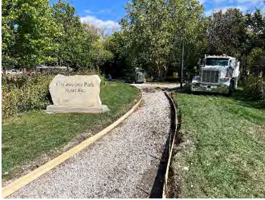
Cornerstone Park concrete trail removal and replacement.
