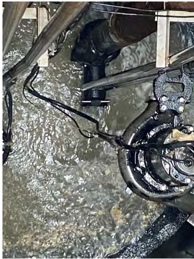
Progress Park Lift Station – Pump pulled and inspected
