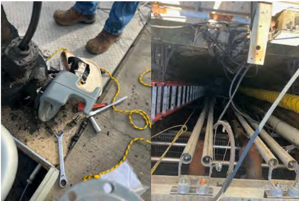
WAS Pump Repairs – Replacement pump base elbows and pump brackets
