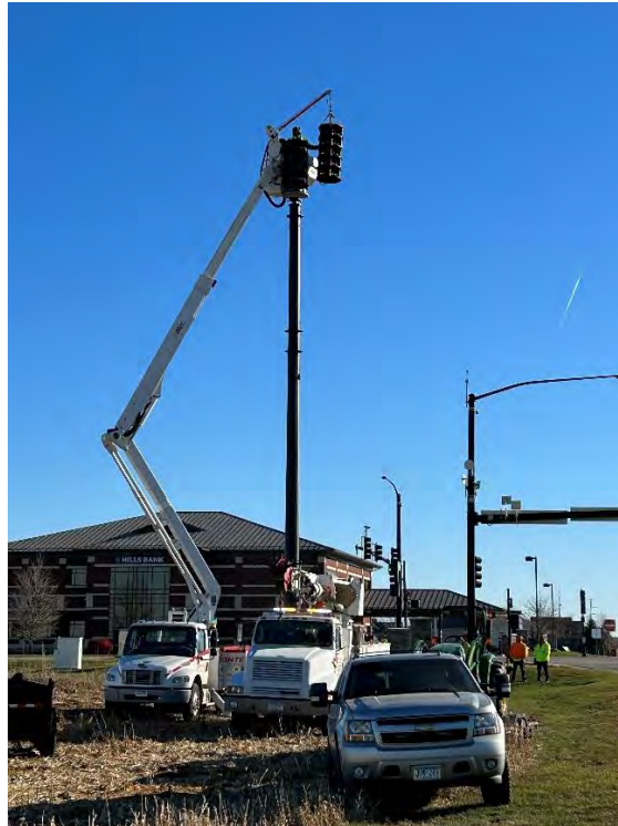
New warning siren being installed
