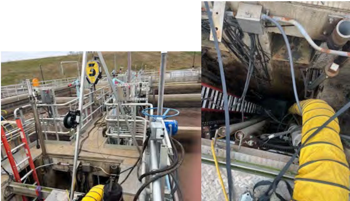
WAS Pump Repairs – Confined Space Setup
