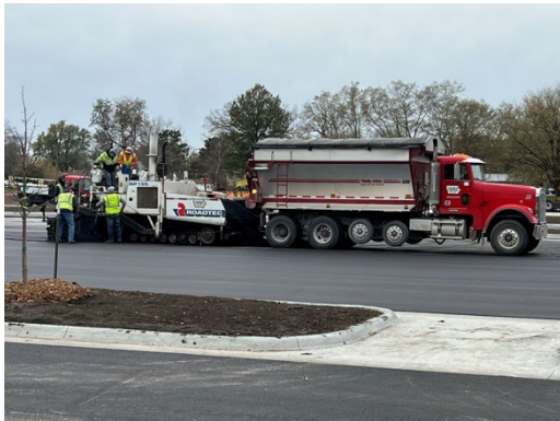
Penn Meadows Park Parking Lot project receives the final asphalt overlay.
