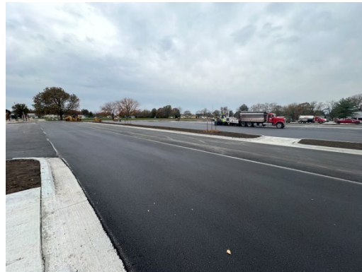
Penn Meadows Park Parking Lot project receives the final asphalt overlay.
