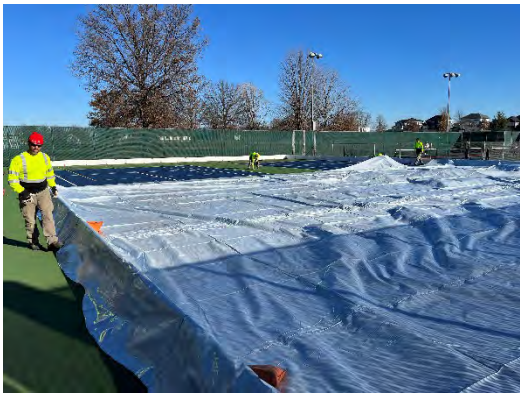
Ice rink installation.
