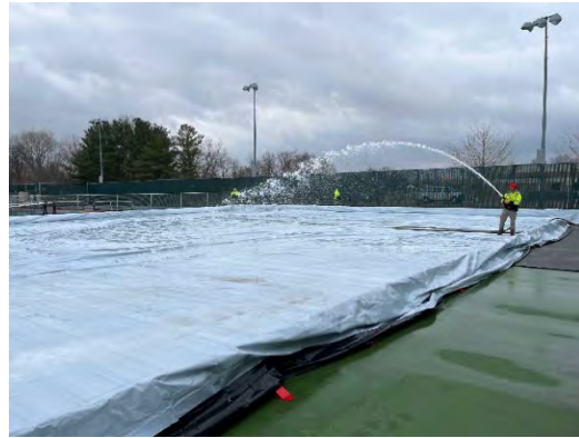
Ice rink installation.
