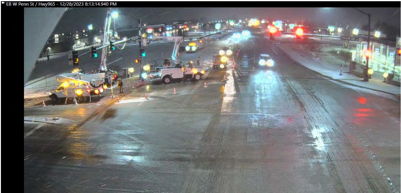
Temporary traffic signal installation
