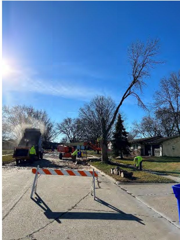
Tree removal in ROW
