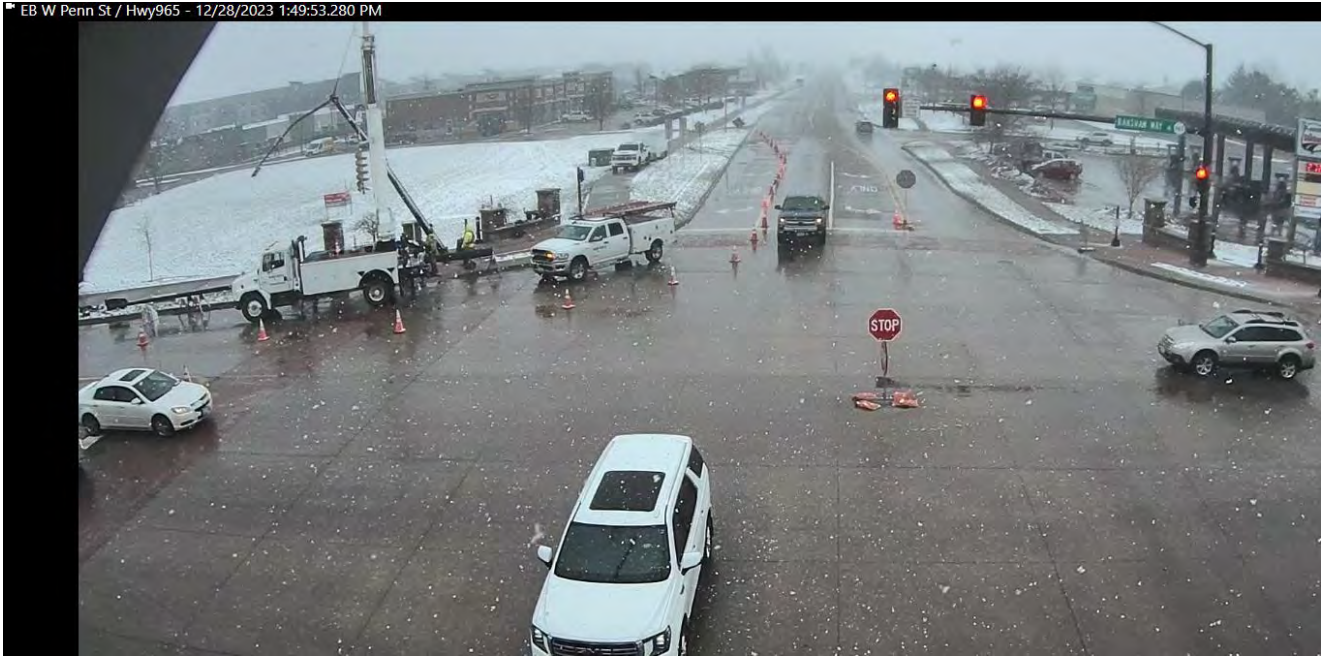
Removal of damaged pole
