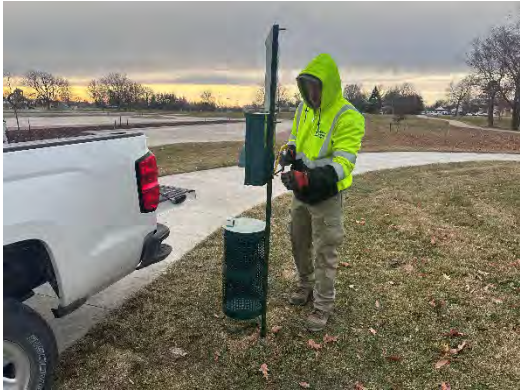
Pet Waste Station installation.
