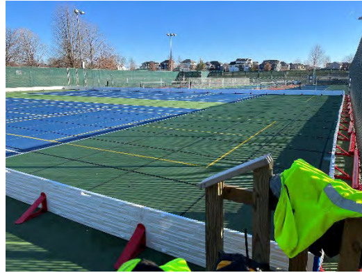
Ice rink installation.
