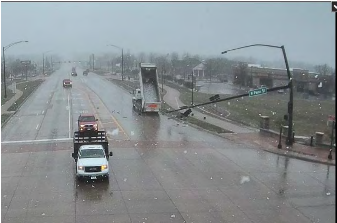
Damaged southbound traffic signals
