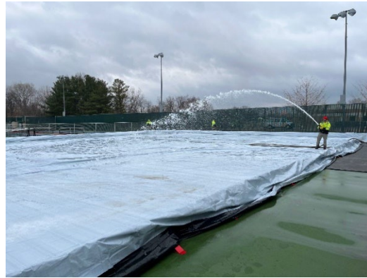
Ice rink installation.
