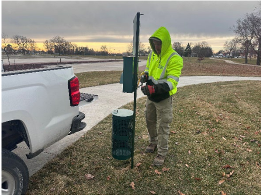
Pet Waste Station installation.
