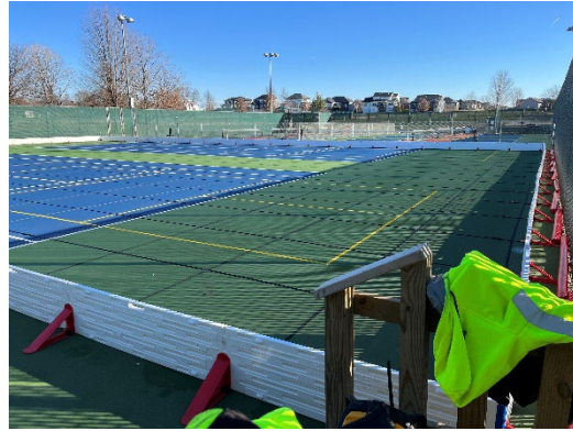
Ice rink installation.
