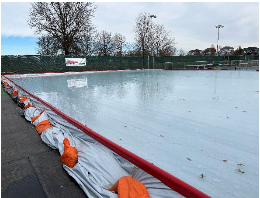
Finished ice rink installation.
