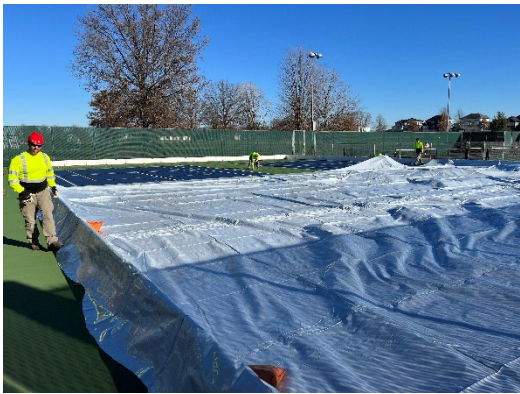
Ice rink installation.
