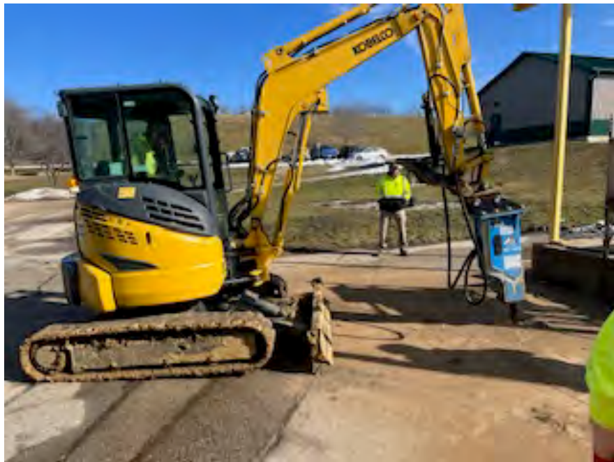
Removal of Asphalt
