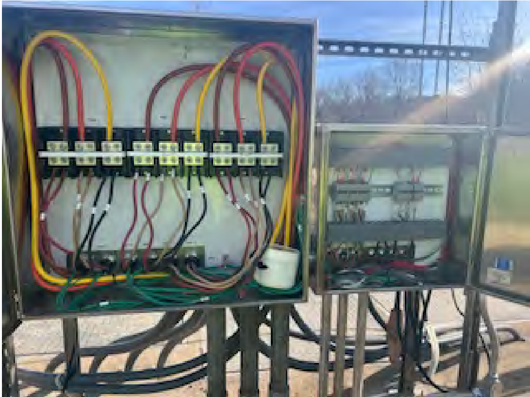
New Pump Control Wiring
